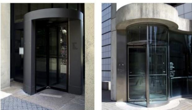
Figure 2. Revolving doors at MIT Campus with hidden swing doors.
