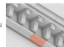
Architrave 3/71 cracked 4/71 spalled 1/71 missing
