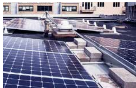
Marcus Garvey Village, Solar + Storage Installed by: Demand Energy
