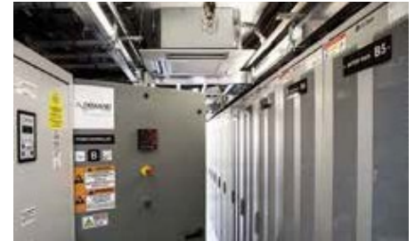
Marcus Garvey Village, Solar + Storage Installed by: Demand Energy
